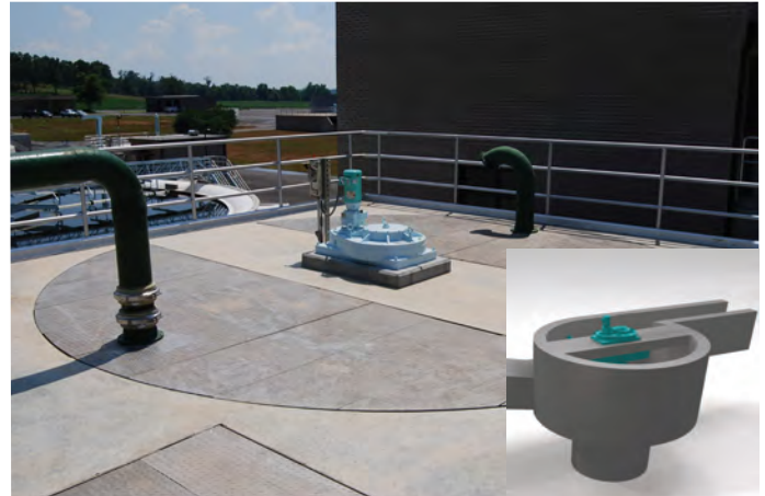
An exterior view of the Rogers PISTA® 360™ grit removal system.
