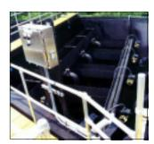
S&L provided two complete **NUTRIGEST®** wastewater treatment systems to allow for future considerations and effluent reuse for irrigating a nearby golf course. This **NUTRIGEST®** system contains multiple treatment zones, an inner secondary clarifier (lower left) and tertiary filter cells (lower right) which work to provide high-quality effluent.
