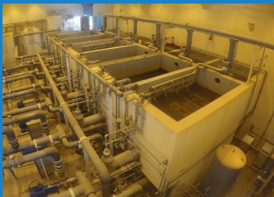
This is a 15 MGD Cerafiltec retrofit installation of a polymeric membrane treatment system.
