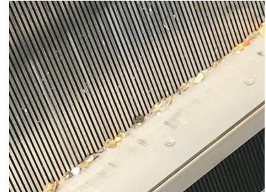
This 2 mm screen will dramatically improve the downstream plant O&M.
