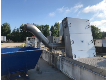
Or-Tec Micro Bar Screen and Swan Neck Compactor
