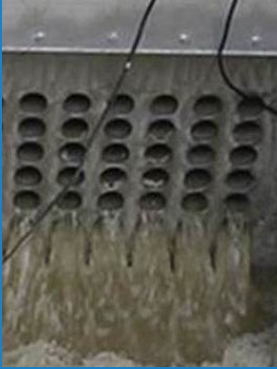
Flow pacing allows for bulbs to be turned off when flow is low.
