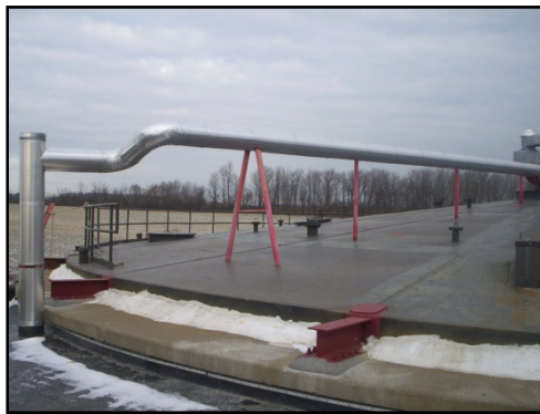
Figure 1 Welded Secondary Digester Cover
