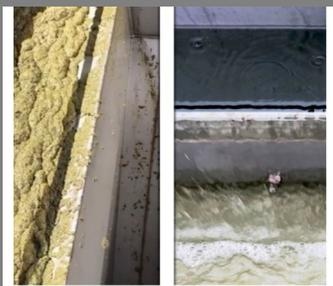
*The froth created by the SAF is comprised of bubbles (7 to 25 microns) that have an electrically-charged surface and greater surface tension. This gives them higher solids capture rate and removal.*
